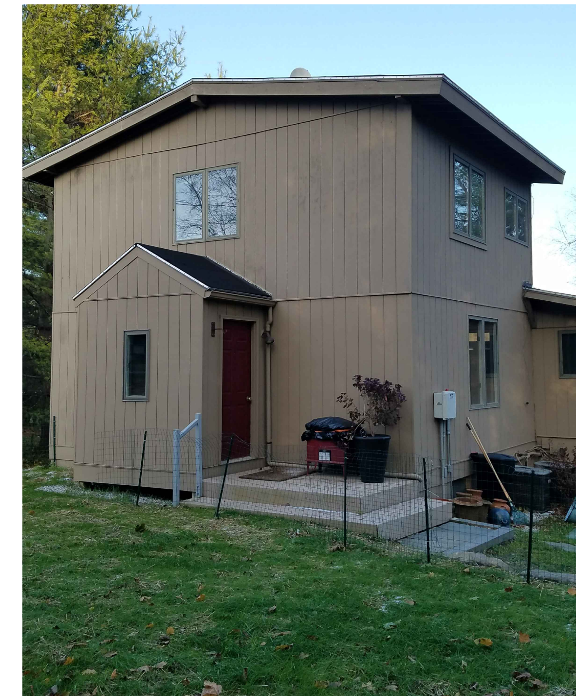
3 EXISTING WEST EXTERIOR PHOTO NOT TO SCALE
