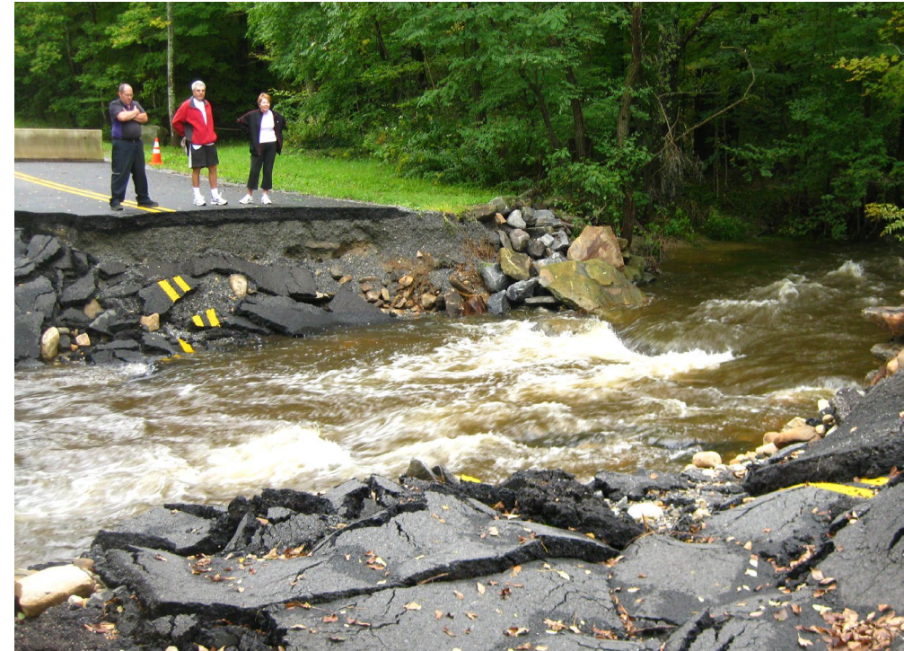
Failure of Benton Hill Culvert
