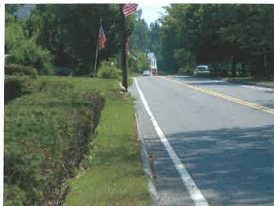
Photo 4: Rt. 23 East—1-foot shoulder on north side of road
