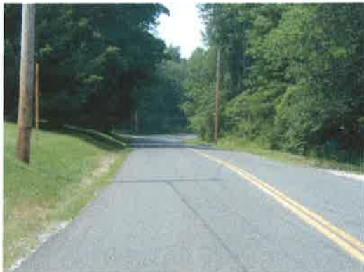
Photo 1: Blue Hill Road looking North
