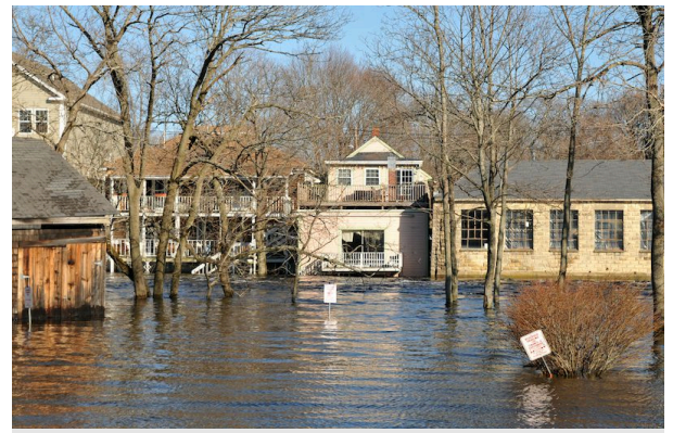
Flooding along the Ipswich River
